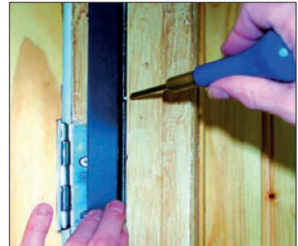
Step 3: Panel pins finish
